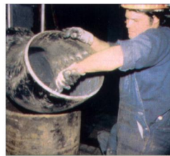
Repair/Line Cold Pipe Elbows with Wear Guard High Load
